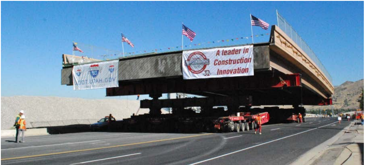
Figure 2: SPMT transporting a bridge superstructure
