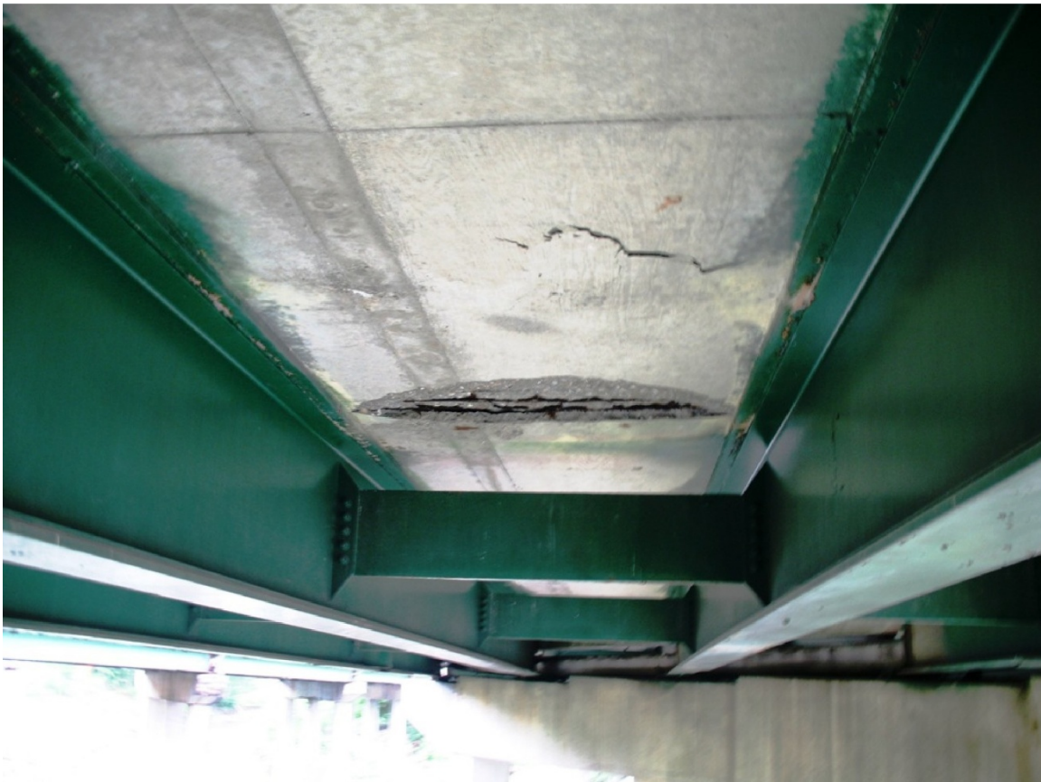
Deck Issues as Seen from Below and Relatively Good States of Beams
