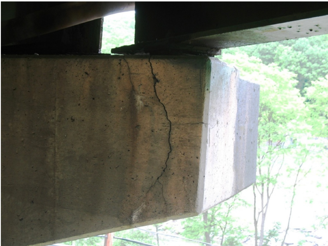
Pier Cap Distress under Exterior Beams
