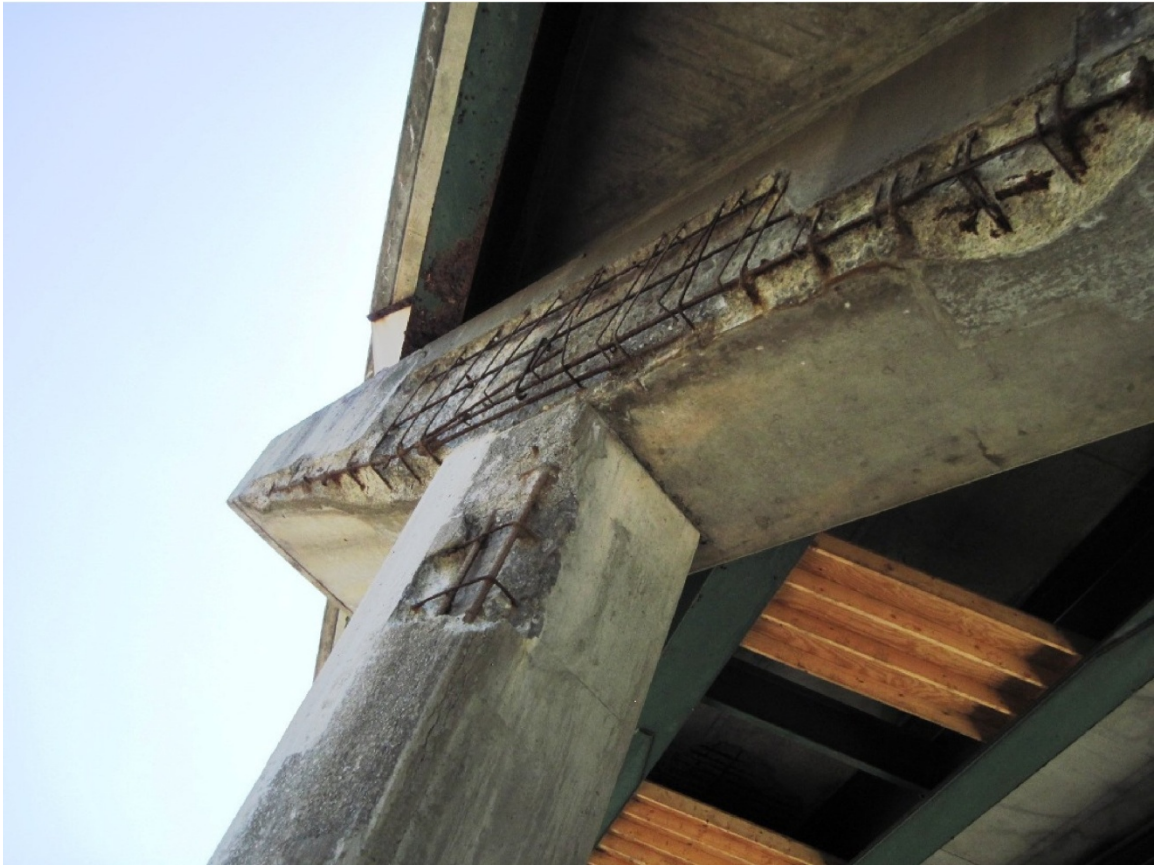
Pier Cap Deterioration Caused By Leaking Joints
