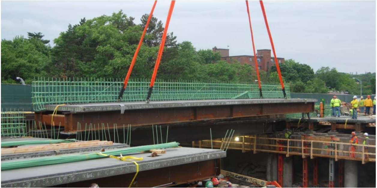
Figure 3: PBU being lifted into place
